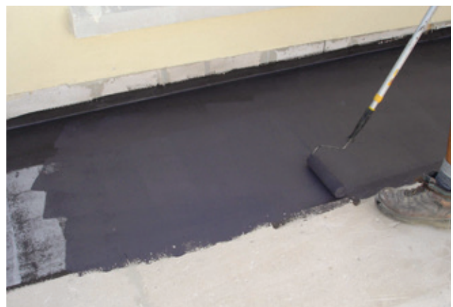
Applying second coat of AtomX™ Tanking Membrane over AtomX™ Tanking Mesh.
