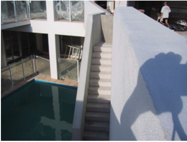
Exterior Stairs before Coating.
