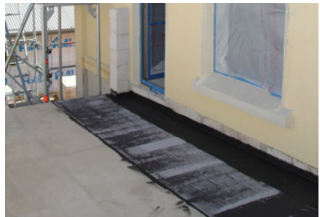
A deck with AtomX™ Tanking Mesh pressed into first coat of AtomX™ Tanking Membrane.
