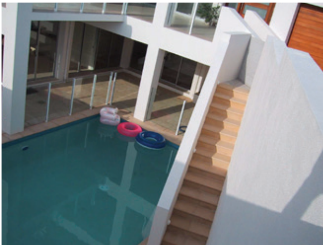
Finished Exterior Stairs.
