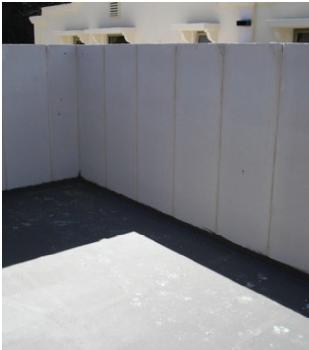
A deck showing AtomX™ Tanking Membrane up dividing wall and tiles partly laid.
